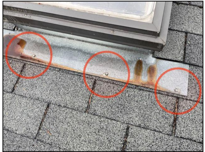
Exposed fasteners
