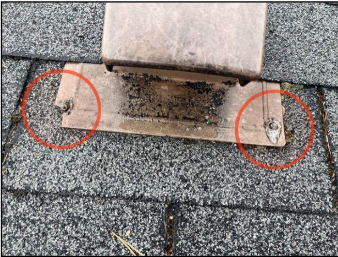
Exposed fasteners
