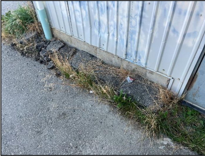
Improper drainage
