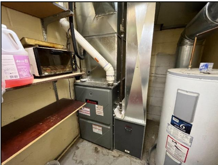
Gas-fired, high-efficient
