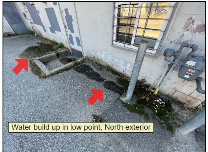
Improper grading
