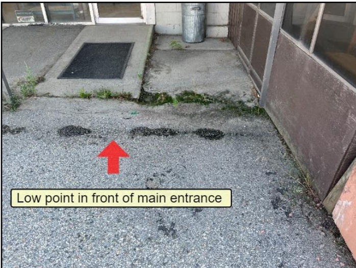
Improper grading
