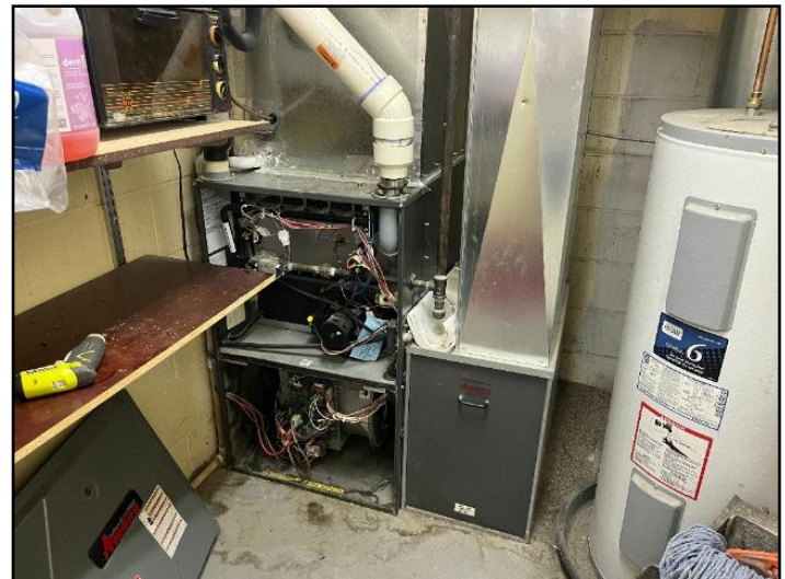
Gas-fired, high-efficient
